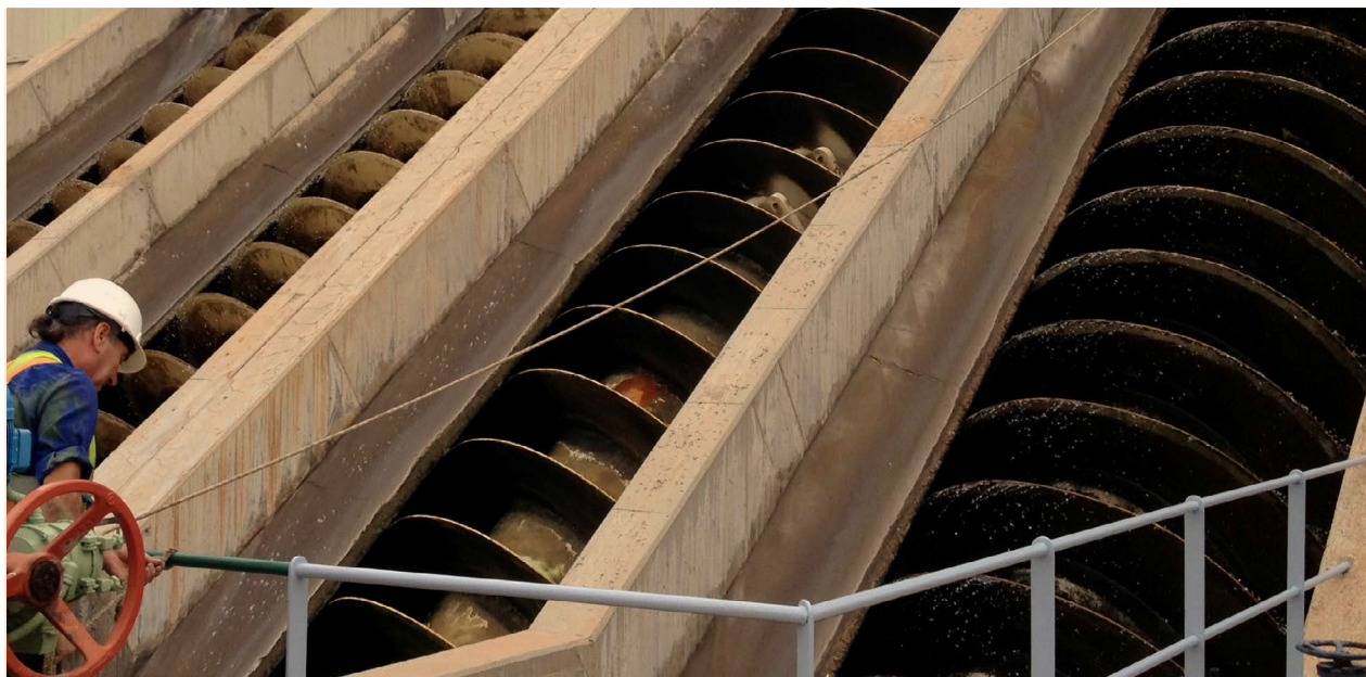
Climate change poses a threat to urban infrastructures, such as treatment plants where the increase in torrential rainfall could outstrip their capacity.
