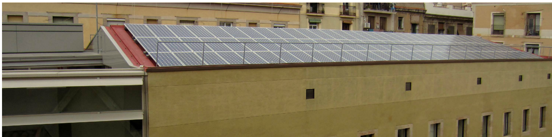
A lot of municipal facilities take advantage of the building's roof to install photovoltaic panels to produce electricity.
